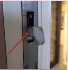
Clean and lubricate moving parts. Use a suitable acid-free oil. This should be done as needed, but at least once a year.
