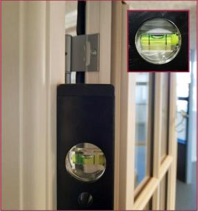
The frame in the hinge side and bottom frame must be plumb and level. Air/clearance between sash and frame must be the same all the way around.
