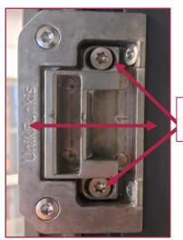
Loosen screws and adjust insert
