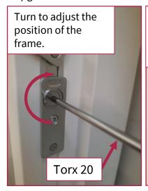
When the mark is pointing down, the frame is adjusted as high up as possible.
