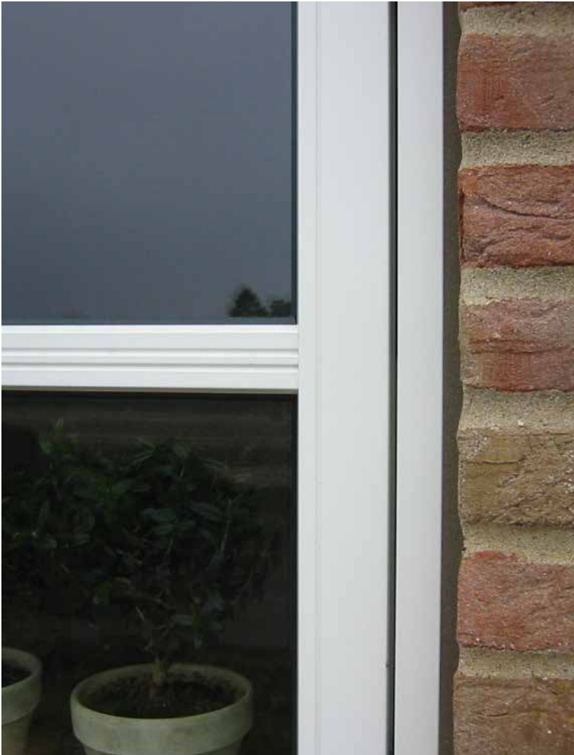
Cottage window with modern energy saving aluminum glazing bars
